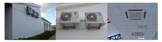
Figure I.2.3.25 Newly renovated cooling and heating system in the E 1 and 2 block studios
